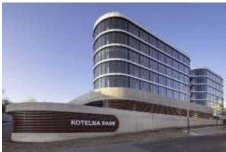
[Kotelna Park II CZ.jpg]
